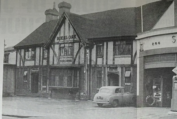
The Royal Oak in the 1950s. Nextdoor was South Bucks Garage which sold petrol from its 'power' pumps.
